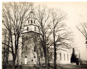
St. Peter's Lutheran Church, built 1786, known locally as Stone Church
