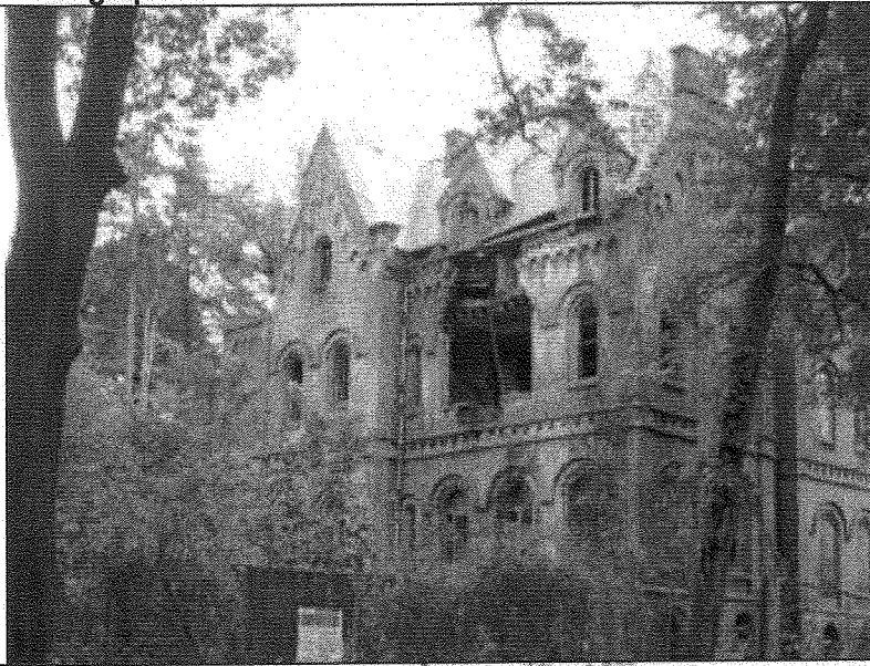
Photo #1: North Facade of House
